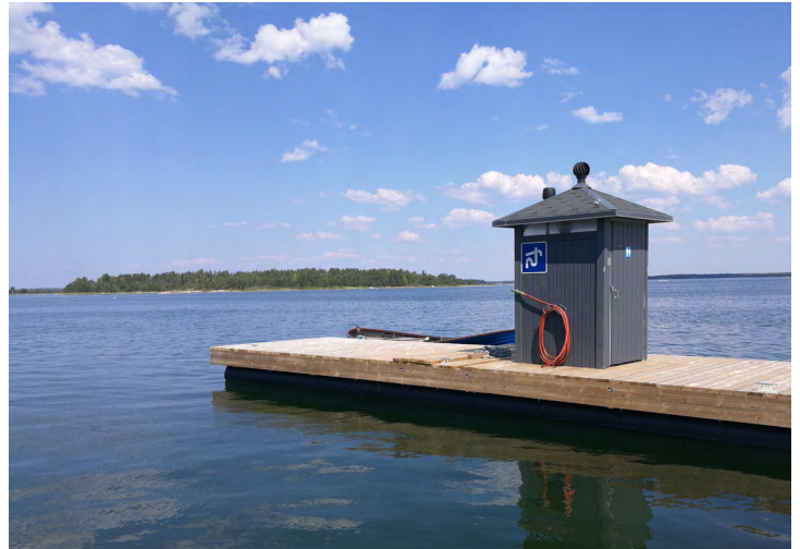
Transportable septic wastewater emptying system in Kuuskajaskari island in Rauma. Photo by Minna Keinänen-Toivola.
