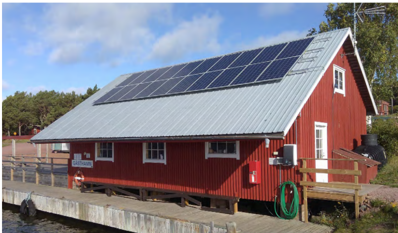
Solar panels in Sottunga port. Photo by Kristiina Kortelainen.
