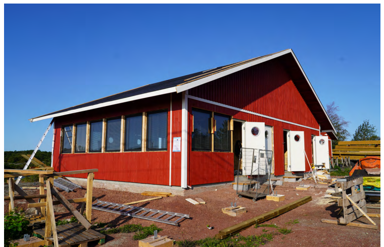
New service house under construction in Kökar Havspaviljongen. Photo by Alberto Lanzanova.
